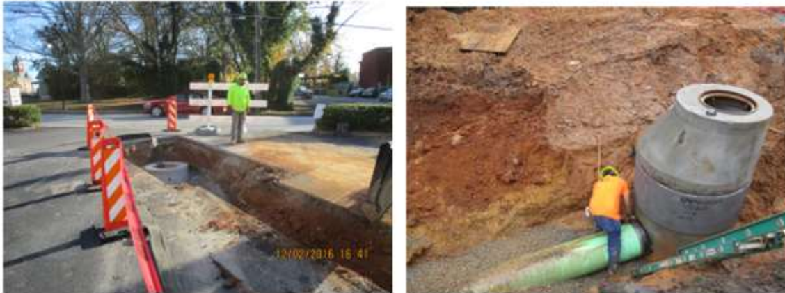
EXHIBIT 2 – Typical Open Cut Gravity Pipe Projects
