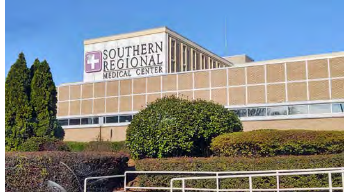
Image Caption: View of Southern Regional Medical Center (2023)
