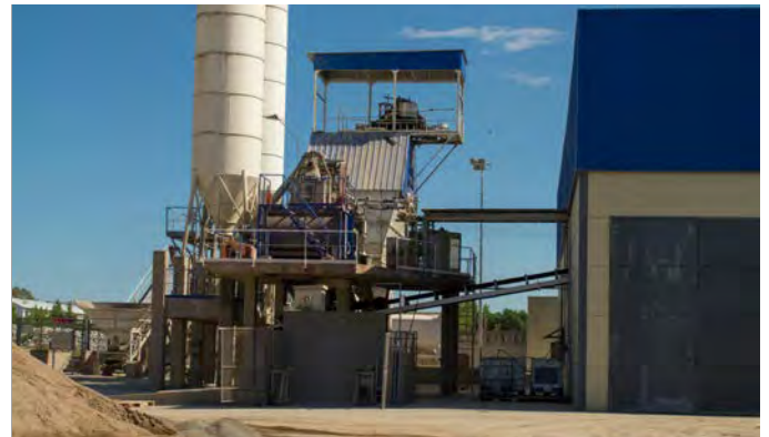
Image Caption: View of industrial plant Source: Mica Asato (2018)
