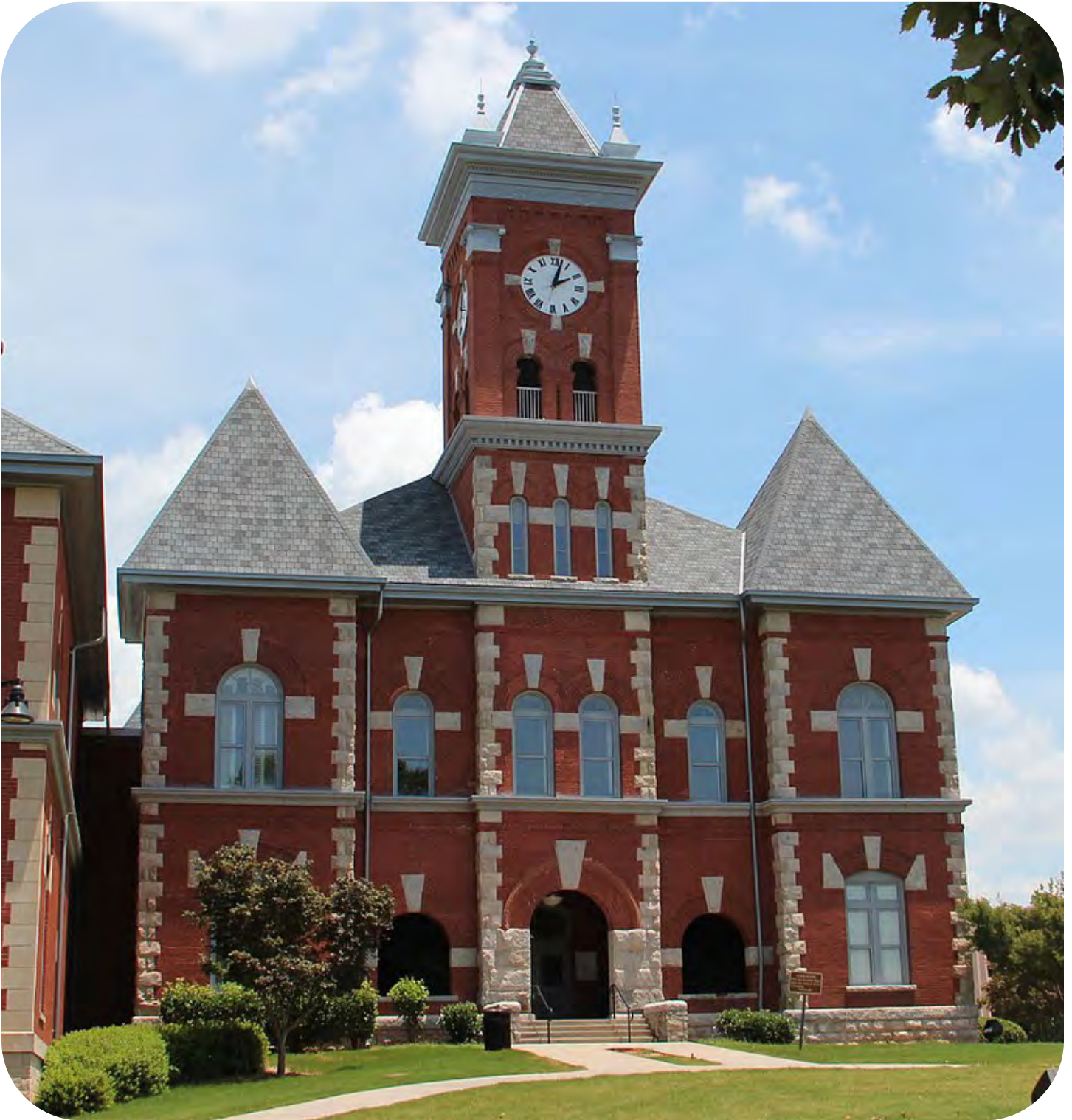
Image Caption: View of Clayton County Courthouse in Jonesboro Historic District Source: Thomson200 (2015)
