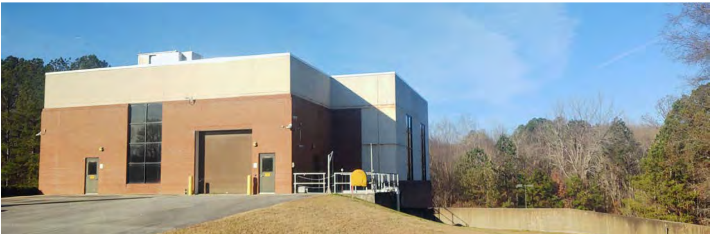
Image Caption: View of Clayton County Water Authority facilities (2024)
