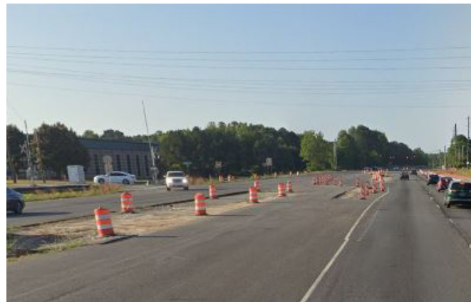
Recent Improvements on Bonanza Segment
