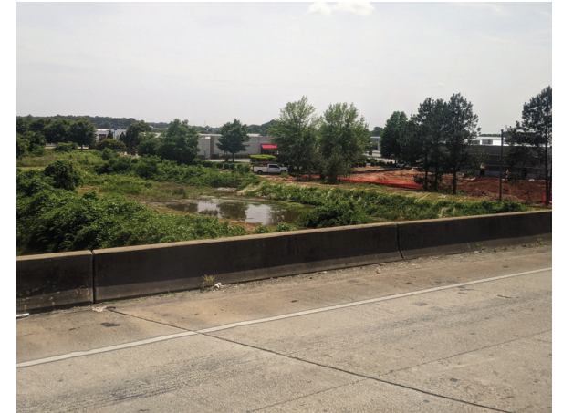
Lack of Sidewalk on Bridge Crossing
