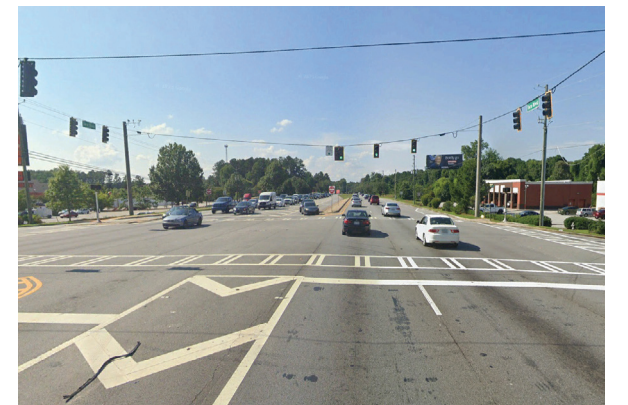
Pedestrian Crossing on a 6-Lane Road
