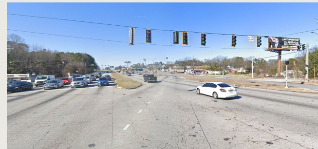
Overwhelming, unsafe interchange of Tara Boulevard + Old Dixie Rd (provides 8 lanes of travel)
