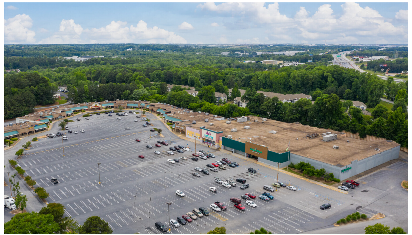
Overhead view of existing conditions on site
