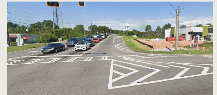
Primary entrance to downtown Lovejoy is narrow and only provides vehicular access
